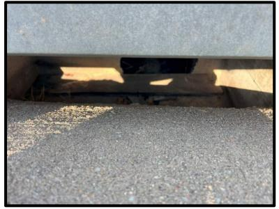
Picture 15: Erosion at Drainage Basin – 8/28/2024
