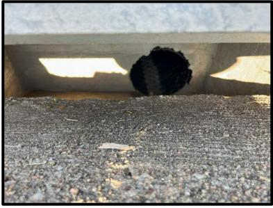
Picture 16: Erosion at Drainage Basin – 8/28/2024
