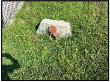
Picture 12: Downspouts on East Side of Main Building – 8/28/2024
