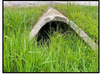
Picture 20: Culvert Inlet Separation Northeast of Facility – 8/13/2024
