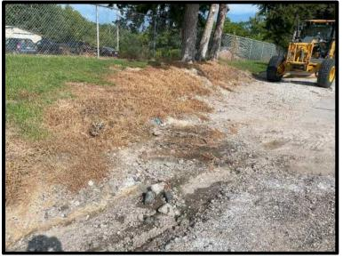
Picture 34: Embankment Washout along West side of Facility – 8/27/2024
