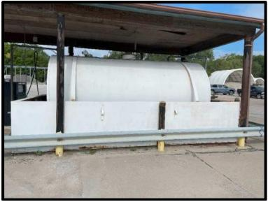
Picture 2: Rusting at Base of East Side Diesel Secondary – 8/27/2024
