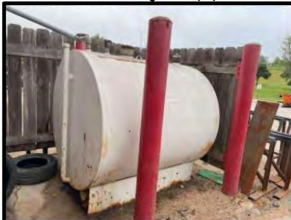
Picture 14: Outdoor Used Oil Storage Tank – 8/13/2024
