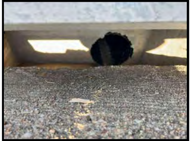
Picture 16: Erosion at Drainage Basin – 8/28/2024
