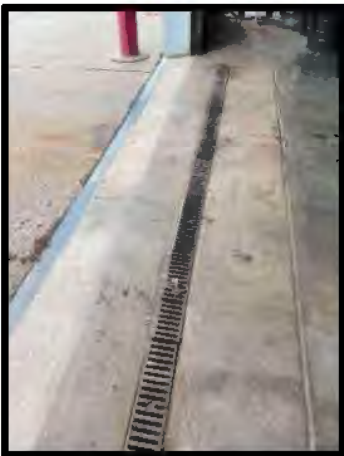
Picture 31: Indoor Trench Drains and Berms – 8/13/2024
