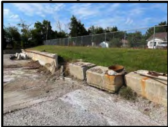
Picture 35: Embankment Washout along West side of Facility – 8/27/2024
