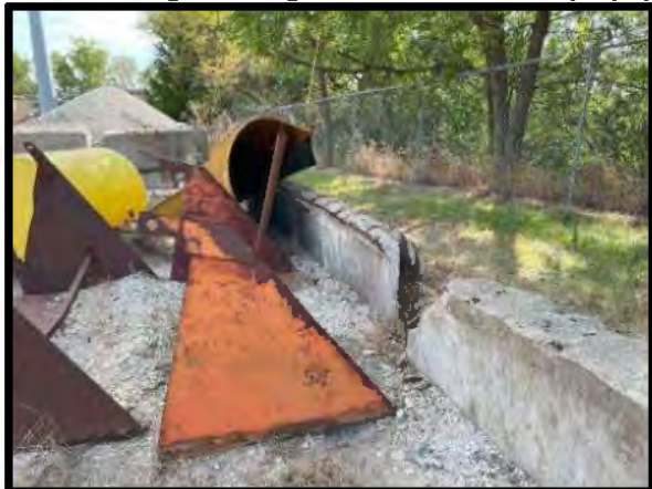
Picture 27: Damaged Retaining Wall Section South of Facility – 8/27/2024
