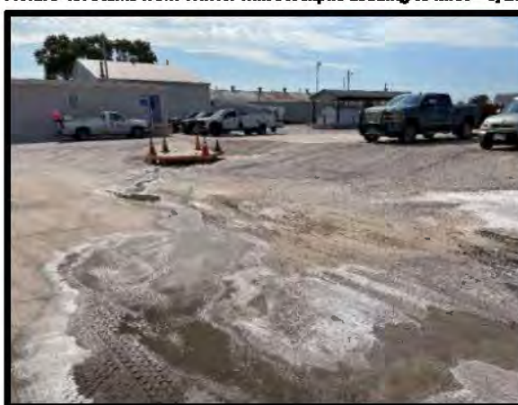
Picture 40: Stains from Winter Mix Stockpile Leading to Inlet – 8/27/2024
