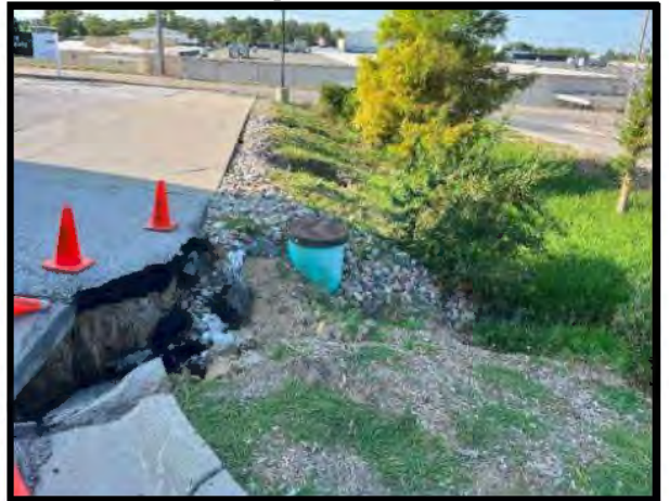
Picture 16: Erosion at Drainage Basin – 8/28/2024
