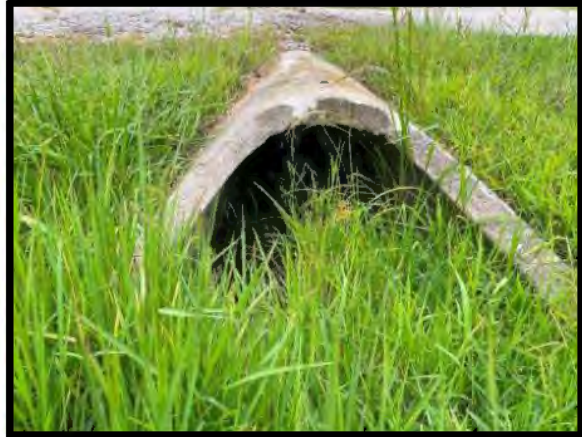
Picture 20: Culvert Inlet Separation Northeast of Facility – 8/13/2024
