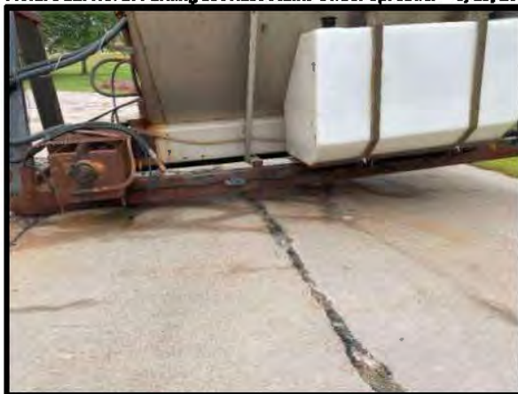
Picture 12: North Parking Lot Rust Stains Under Spreader – 8/13/2024
