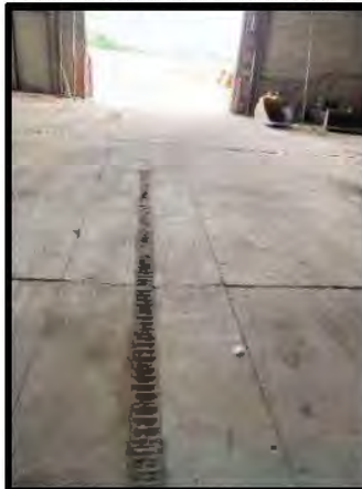
Picture 16: Floor Drain Inside Street Department Storage Building – 8/27/2024
