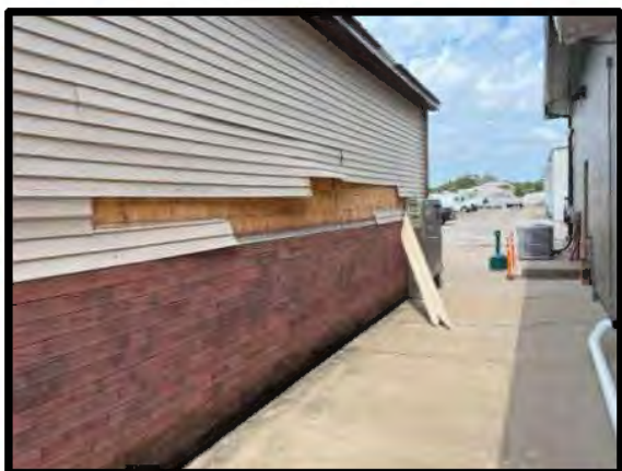
Picture 7: Southwest Garage East Siding Damage – 8/15/2024
