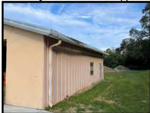
Picture 16: Damaged Gutter on North Side of Lower Equipment Shed – 8/27/2024
