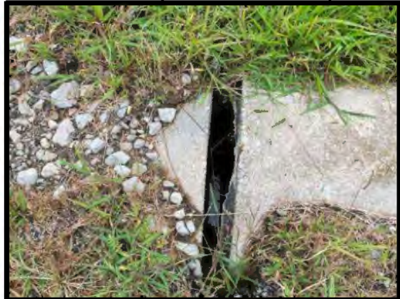
Picture 20: Culvert Inlet Separation Northeast of Facility – 8/13/2024
