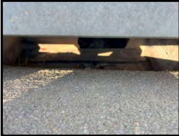
Picture 15: Erosion at Drainage Basin – 8/28/2024
