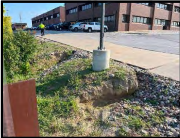
Picture 15: Erosion at Drainage Basin – 8/28/2024
