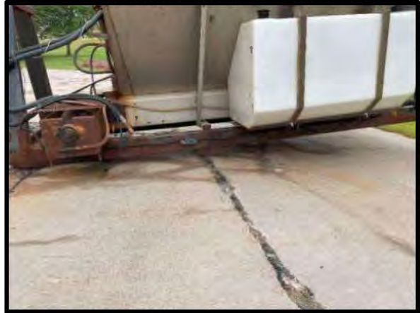
Picture 12: North Parking Lot Rust Stains Under Spreader – 8/13/2024
