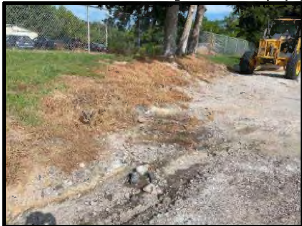
Picture 35: Embankment Washout along West side of Facility – 8/27/2024
