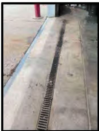
Picture 31: Indoor Trench Drains and Berms – 8/13/2024
