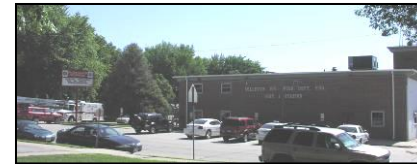
Photo B-27: District 1 Station
