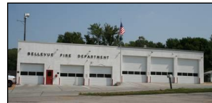
Photo B-28: District 2 Station
