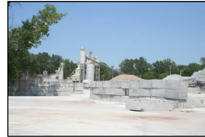
Photo C-32: Concrete Industrial Facility
