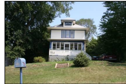
Photo C-20: Older Bellevue Boulevard West House
