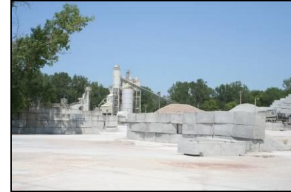
Photo 3-7: The Bellevue Industrial Yard
