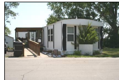
Photo 3-2: A Bellevue Mobile-Home Residence
